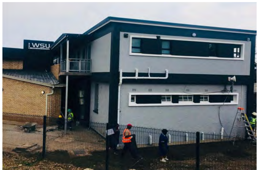
Photo 16: Figure 1 Grey Street Office Space Komani Campus
