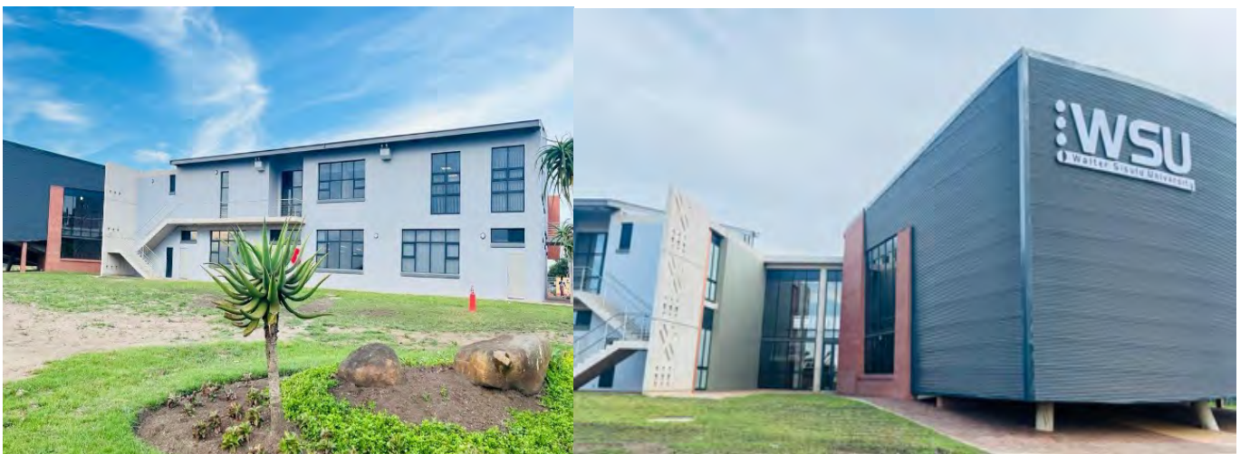
Photos 14: Ibika FMS Building
